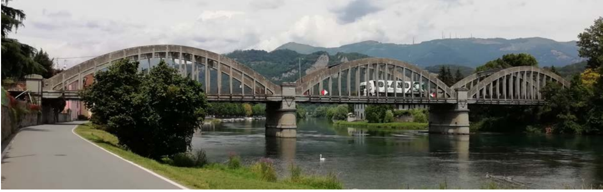
Figure 1: Brivio bridge (1917): downstream view of the road three-span arched bridge crossing the Adda river; Brivio (Lecco) right bank (left), Cisano Bergamasco (Bergamo) left bank (right). Picture taken by author E.R. on 7 July 2022.
