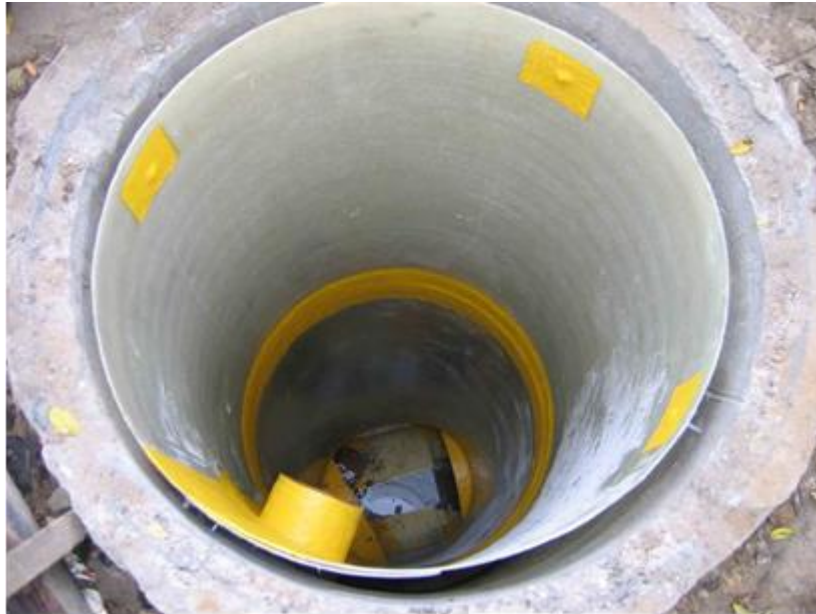
Fig. 4. Renovation method using GRP (TWS) liners
