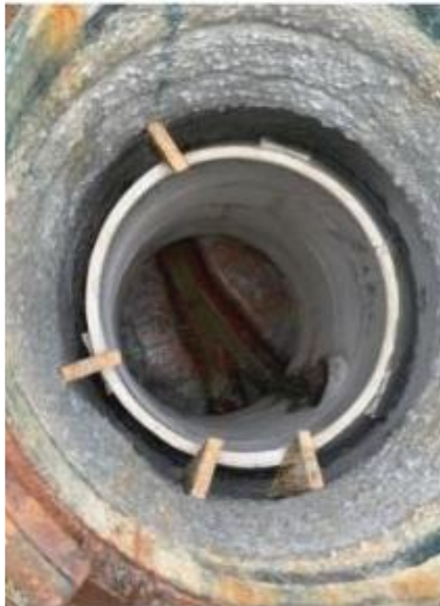
Fig. 5. Renovation method using polymer concrete modules [47]
