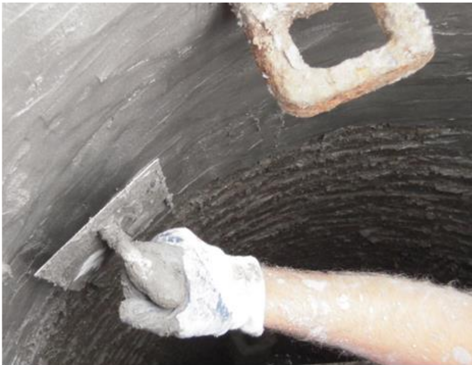
Fig. 7. Restoration of the corroded surface with cement-based materials
