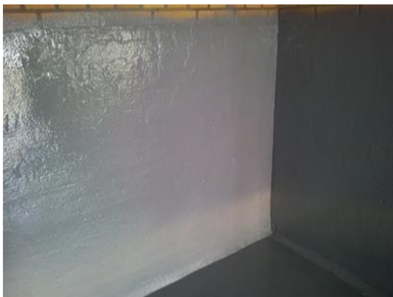
Fig. 3. Renovation method using resins
