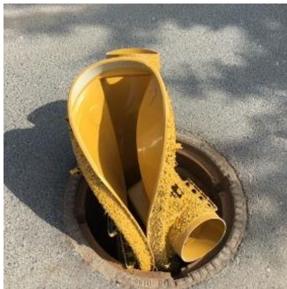
Fig. 6. Renovation method using polyurea liners [48]
